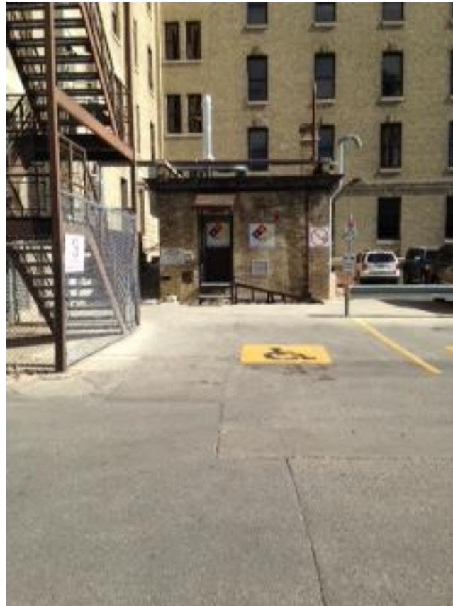
C Block Unloading and Loading Entrance
